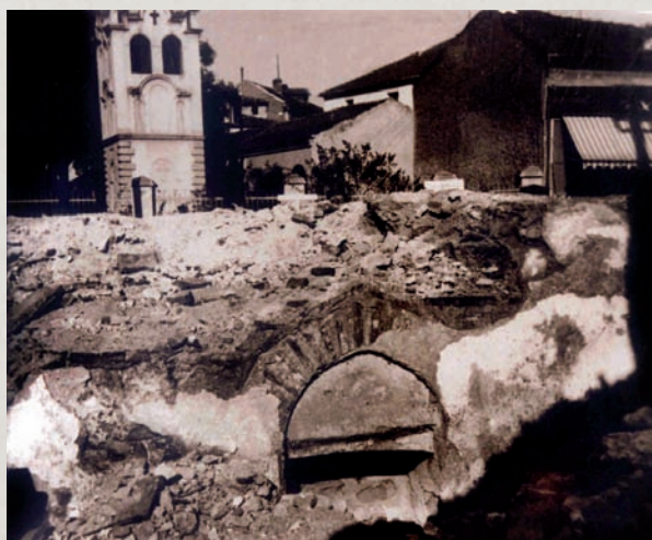
Remains of the mint of Skopje (photo taken after the Skopje earthquake of 1963)
